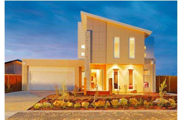
Example of a two-storey home achieving articulation to the street elevation (Portofino by Simonds – www.simonds.com.au )
