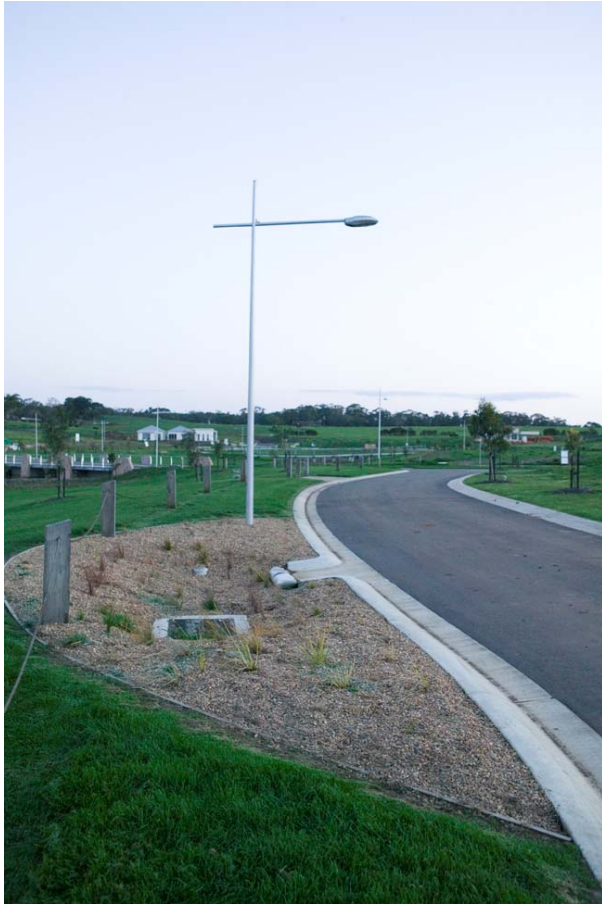
“Rain gardens” are designed to filter stormwater
